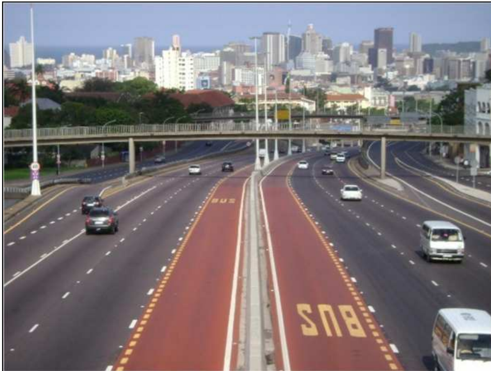
Figure 1: Red continuously graded colourless binder Asphalt on Durban BRT Route 2
