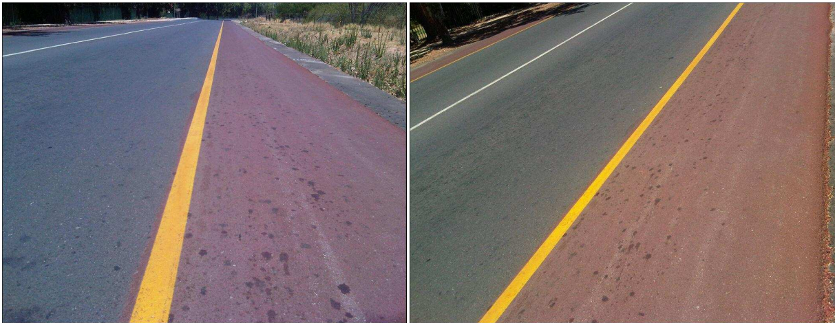
Figure 2: Red Oxide Pigment Coloured Continuously Graded AC Surfacing on Shoulders of R44
