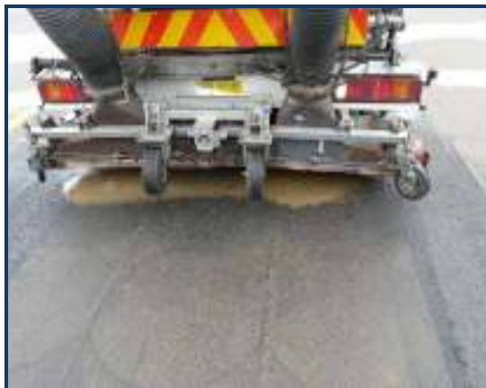
FIGURE 16 : MUDDY SLUDGE EXTRACTED ON LANE 2
